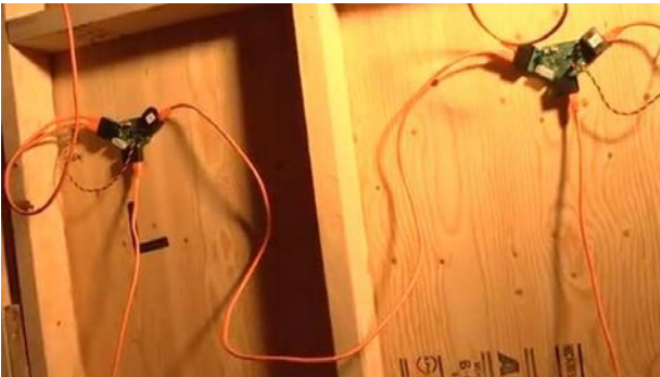
Fig.8 (Top) Plastic pipes and movable coil on the surface. (Bottom) micro-controllers on back side.
